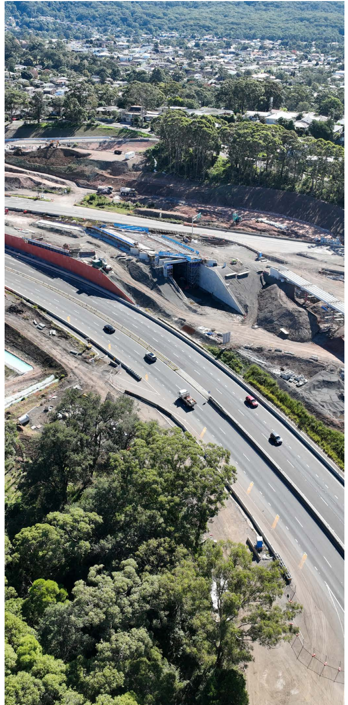
(Above) Mount Ousley Interchange construction Image credit: Transport for NSW
