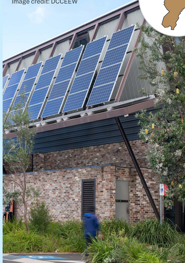
Solar panels on UoW Sustainable Building Research Centre Image credit: DCCEEW
