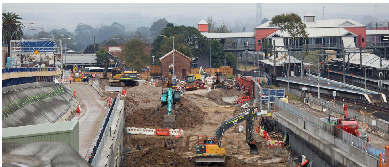
St Marys Metro station, under construction. Image credit: Transport for NSW
