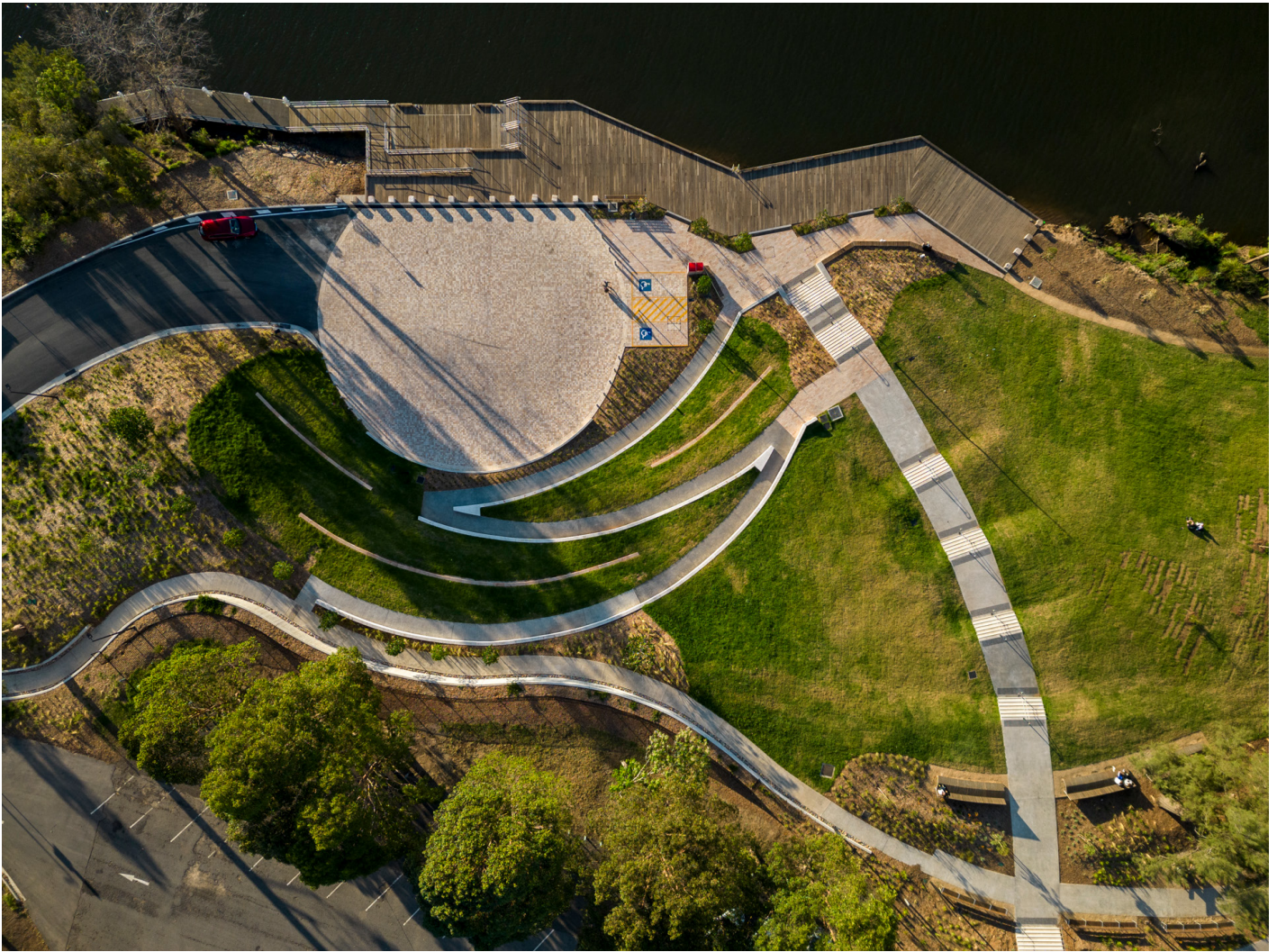
Image 2: Tench Reserve, Penrith City LGA. Completed in 2023 and funded by the Parks for People program.
