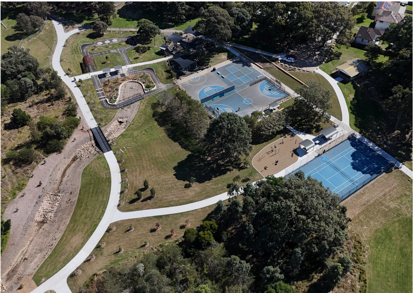
Image 1: George Kendall Riverside Park, City of Parramatta LGA. Completed in 2024 and funded by the Parks for People program.
